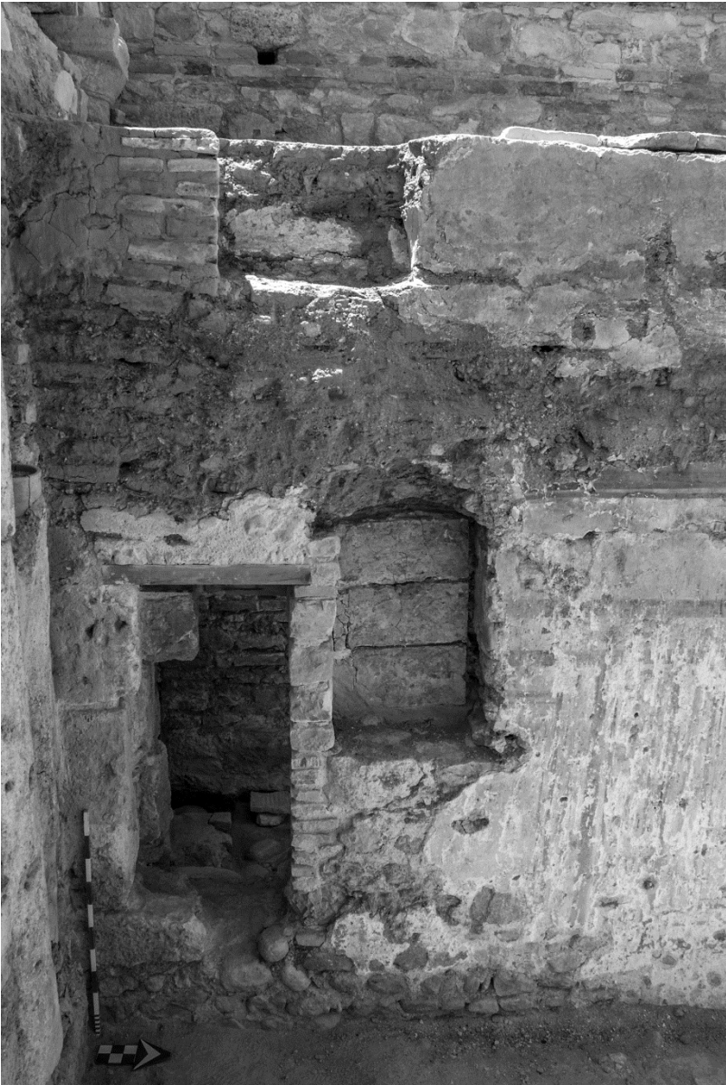
Fig. 14. Taberna 1B, niches of the upper and lower floors.
