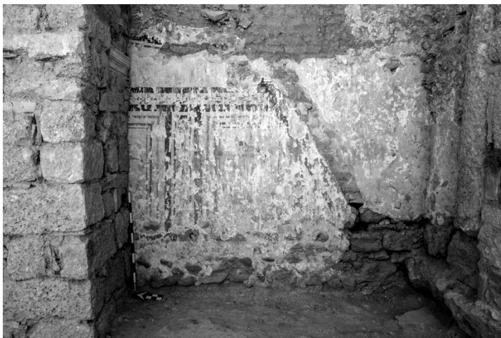
Fig. 12. Taberna 1B, traces of wooden stairs.
