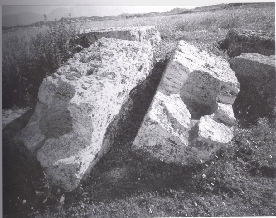
Fig.13: North theatre. Blocks with holes for seating the wooden posts for supporting the velaria .
