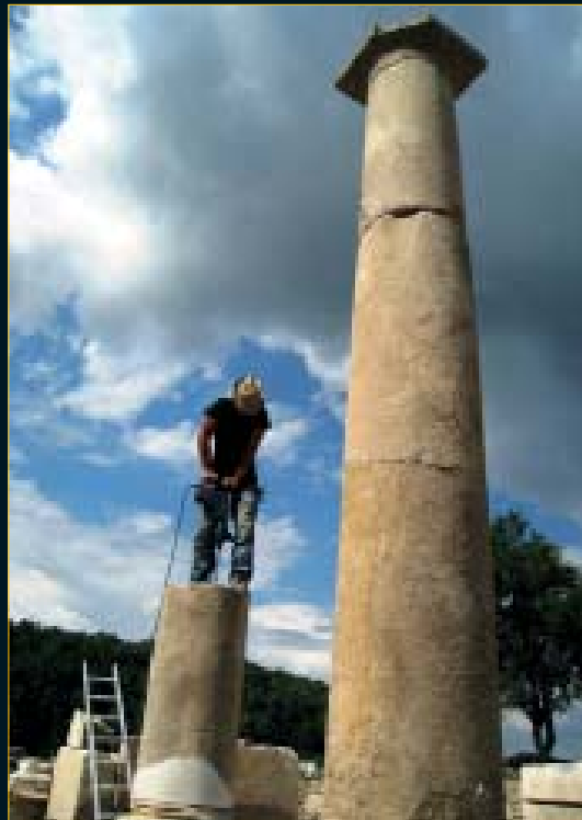
North Road, Restoration works on the columns
