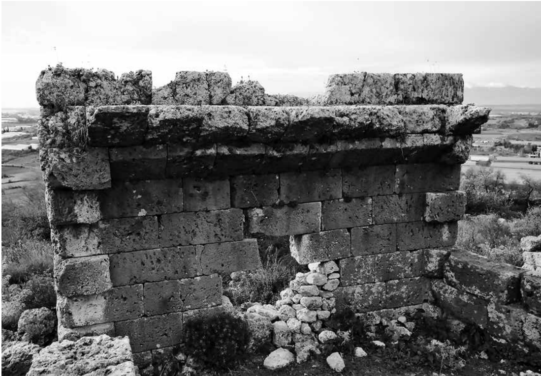
Fig. 14 Tower 1, epalxis on top of north wall
