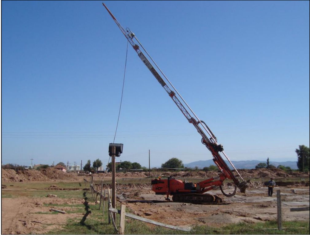
Şekil 4.9: EGT MD1500 Jet grouting delme makinesi (Anonim 2008 a ).
