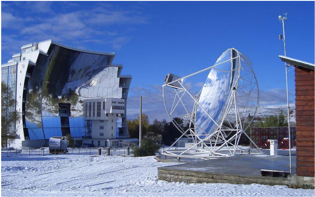
Şekil 3.6: Odeillo, Fransa, 10 kW Çanak/Stirling EuroDish (Sonne SBP, 2020)
