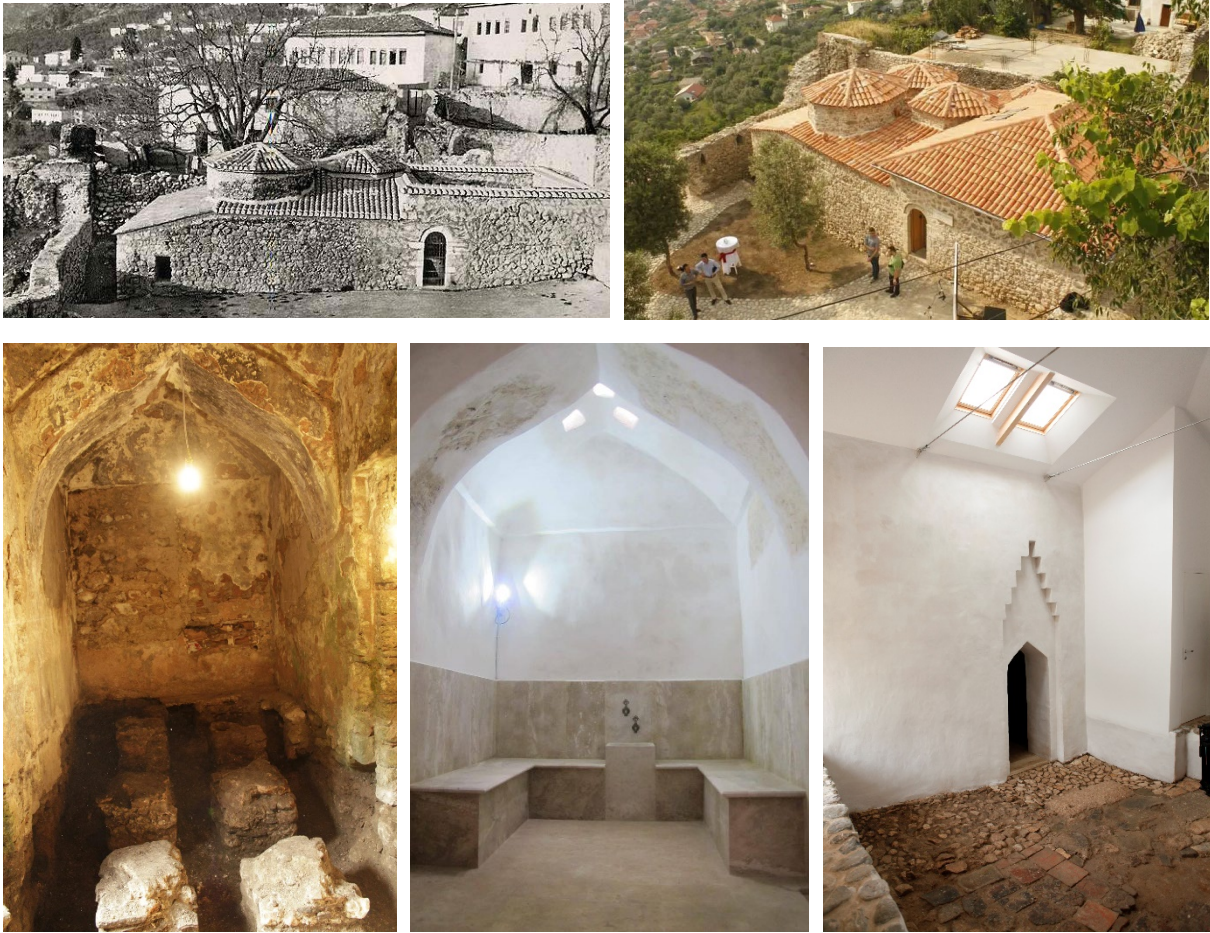
Figure 6 Kruja hamam: 1. Old photo before restoration, 2. Image of the exterior after recent restoration, 3. Interior photo before restoration, 4,5 Interior image after restoration
