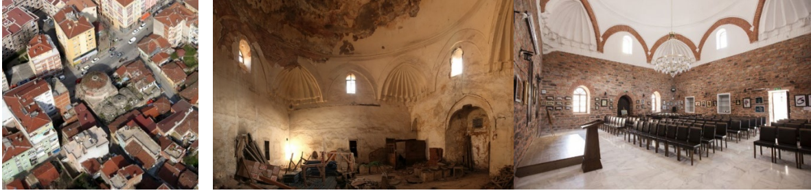
Figure 11 Aerial View, Photo of Incirli Hammam before the Restoration
