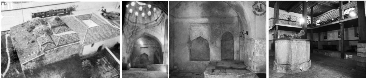
Figure 10 Castle hammam of elbasan: 1,2,3 Image of current interior conditions used as a bar.
