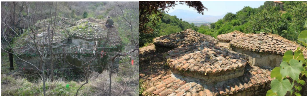
Figure 5 Delvina hamam: 1, 2 Image of existing conditions.
