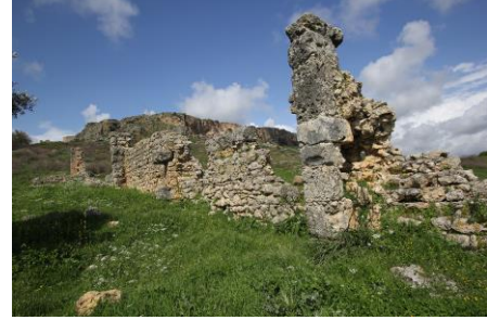
Fig. 14. Aqueduct / Aqueductus , a general view from southwest
