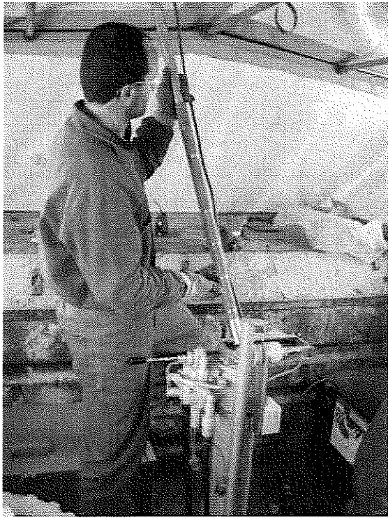
a) Placing ER-VPT tool into hydraulic-push unit
