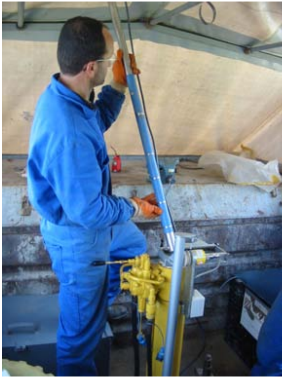
a) Placing ER-VPT tool into hydraulic-push unit
