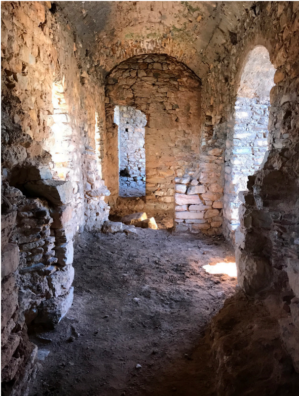
Fig. 14: General view of the south wing looking west: protrusion niches in the front, U04, partitioning walls, U05, doorway opening into U06; after cleaning work (December 2018).
