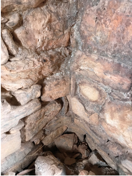
Fig. 13: Joining of the partitioning walls (2018).
