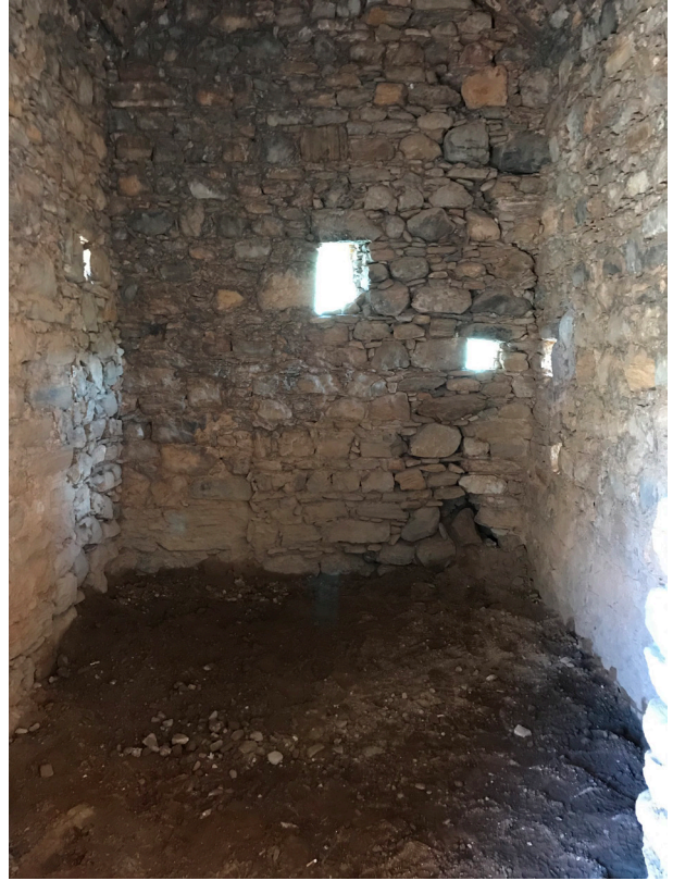
Fig. 11: Unit 03, looking east (2018).
