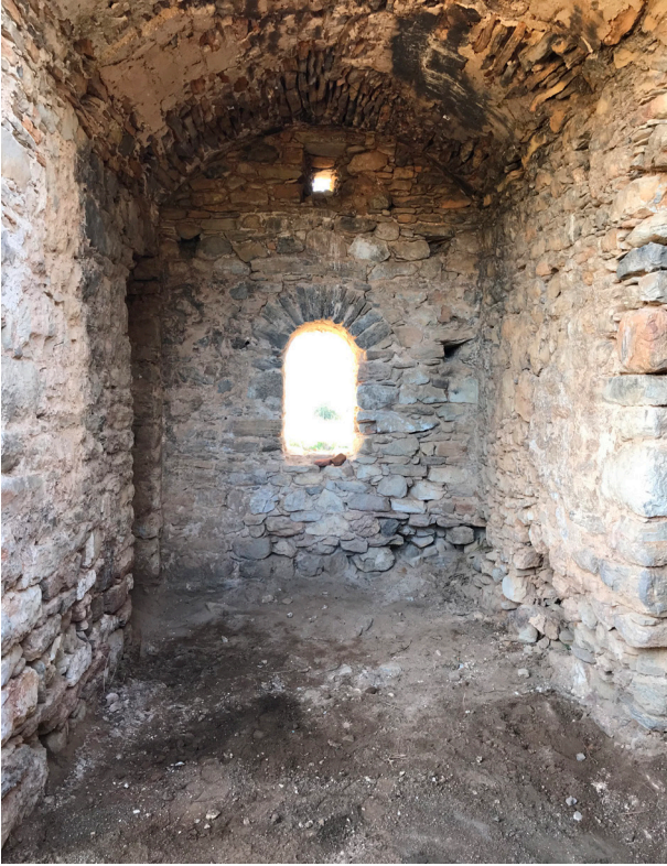
Fig. 18: Unit 06, looking south, after cleaning work (December 2018).
