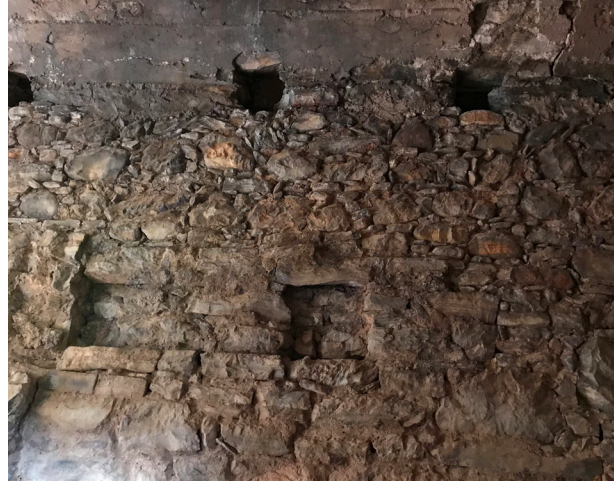
Fig. 21: North wall U03, showing the anomaly and holes for tie beams (2018).
