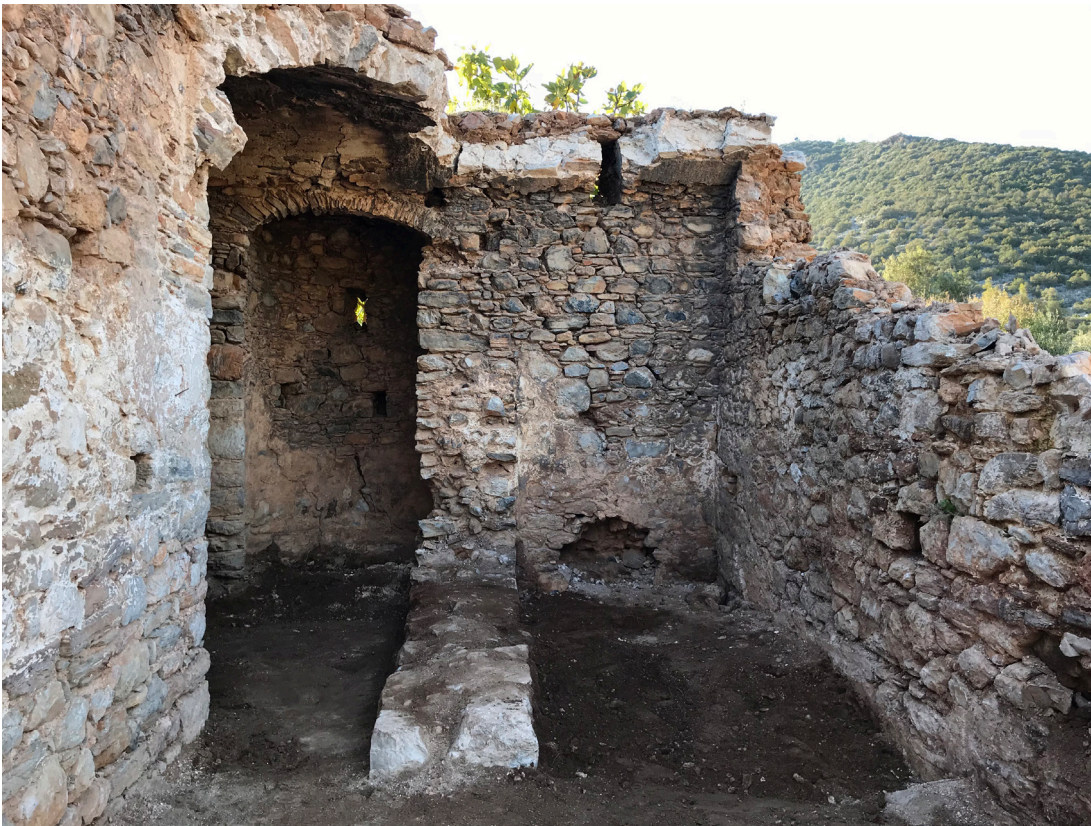
Fig. 17: View of the apse-like protrusion and U07, after cleaning work (December 2018).
