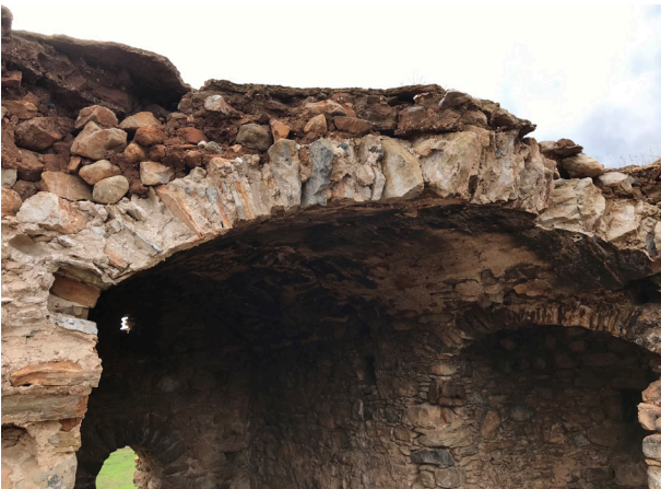
Fig. 6: Detail of the west vault and the mud-stone filling and 'concrete'-like flat roofing (2018).
