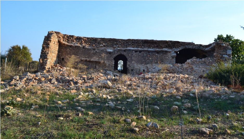
Fig. 2: General view from the north, before cleaning work (November 2018).
