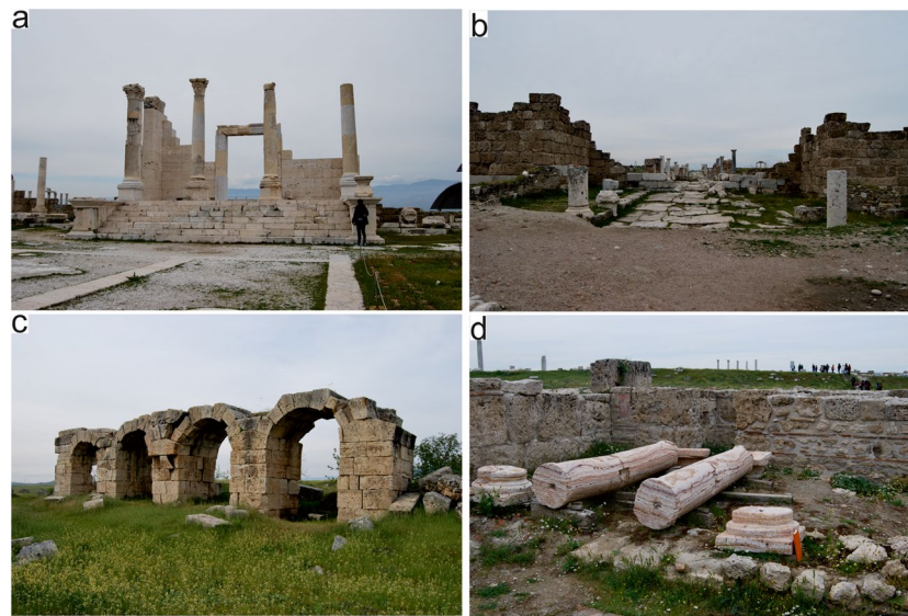
Fig. 7 Some examples on the historical use of the Denizli Travertine at Laodikeia. (a) Temple A, the Laodikeia Ancient City Denizli (photo – Hülya Özen). Mainly travertine blocks and subsequently marble columns have been used, (b) Syrian street, the Laodikeia ancient city, Denizli. The street floor and walls on both sides are made of mostly travertine blocks, but columns along the street and a small
